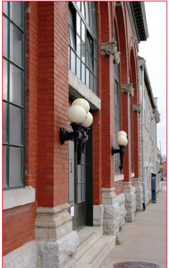
Figure 1: Substation MS1 on Queen Street was the former location of the Kingston Electric Light Company.
